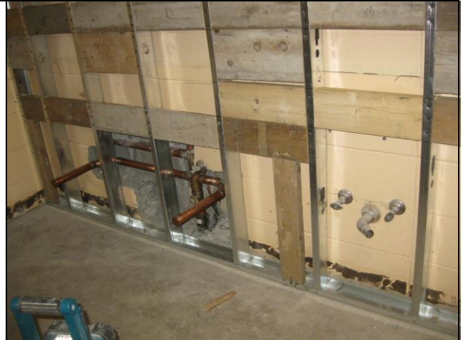
4. Girl's washroom 112 framed plumbing wall
