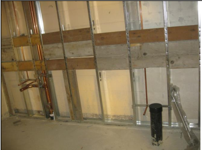
5. Universal washroom framed plumbing wall
