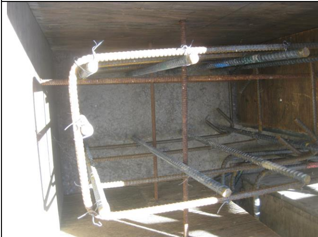
9. Foundation – new classroom
