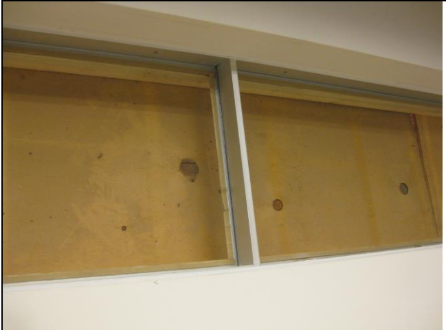
3. Office window frames
