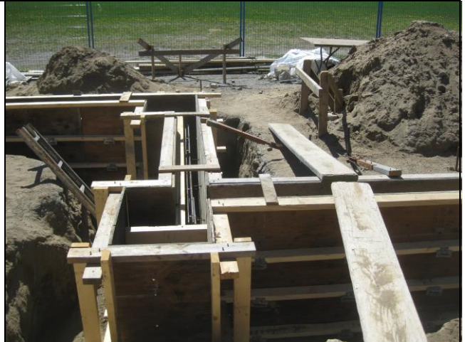
8. Foundation – new classroom
