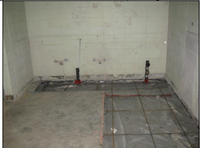
6. Boy's washroom framed plumbing wall
