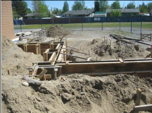
7. Foundation – new classroom
