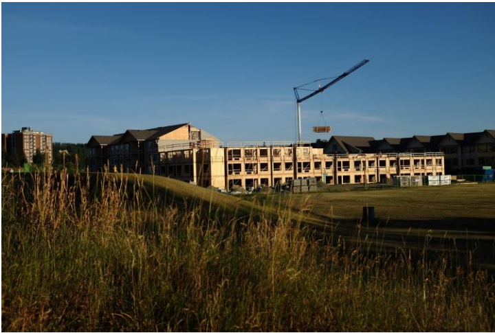
Construction at Riverbend Housing Development
